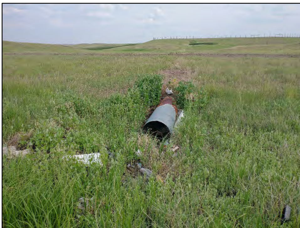
Photograph 16: View of PP-16, existing culvert access road, looking south.
