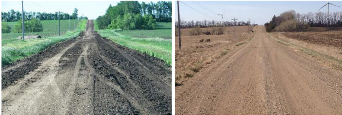
Before/after gravel rehabilitation. Image source: Ken Skorseth, Program Manager, SDLTAP; used with permission
